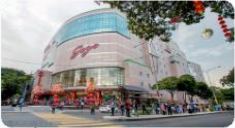
KL Sogo Relamp 1st Phase
