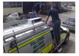
Sensor box installation on vehicle
